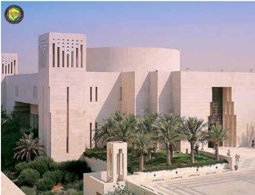
Foto: Courtesy of the GCC Patent Office
