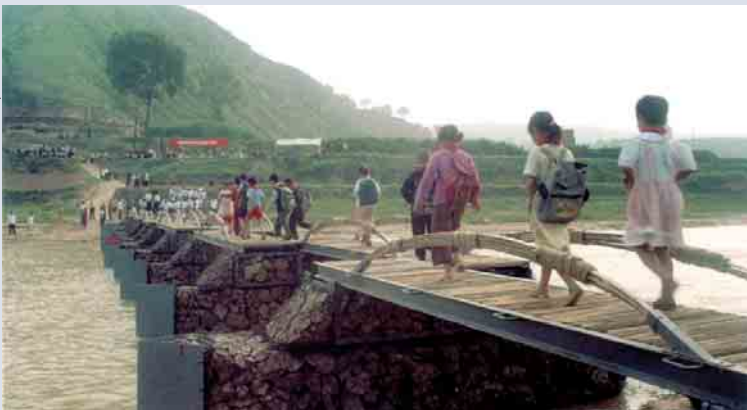
School children from Maosi village in Gansu Province, China, commute safely to school across the bridge that they helped build.
