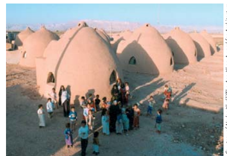
Depending on the external finish, the domes can be either temporary refugee shelters or homes lasting up to 30 years.
