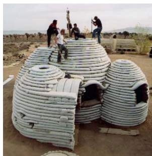
Depending on the external finish, the domes can be either temporary refugee shelters or homes lasting up to 30 years.
